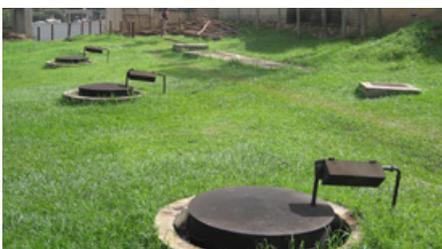
Visit to 4 biodigesters in parallel digesting the waste-water and faecal sludge from the Rubaga Hospital, Kampala, Uganda (November 2014). © J.-M. Médoc
