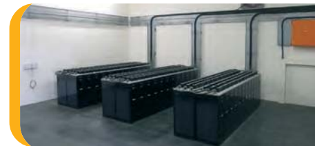
Very well designed and looked after ROOISAND Desert Ranch's hybrid power system. The picture shows the battery bank room with space for growth (currently 6,000 Ah battery capacity at 48 V) [Source: THI]
